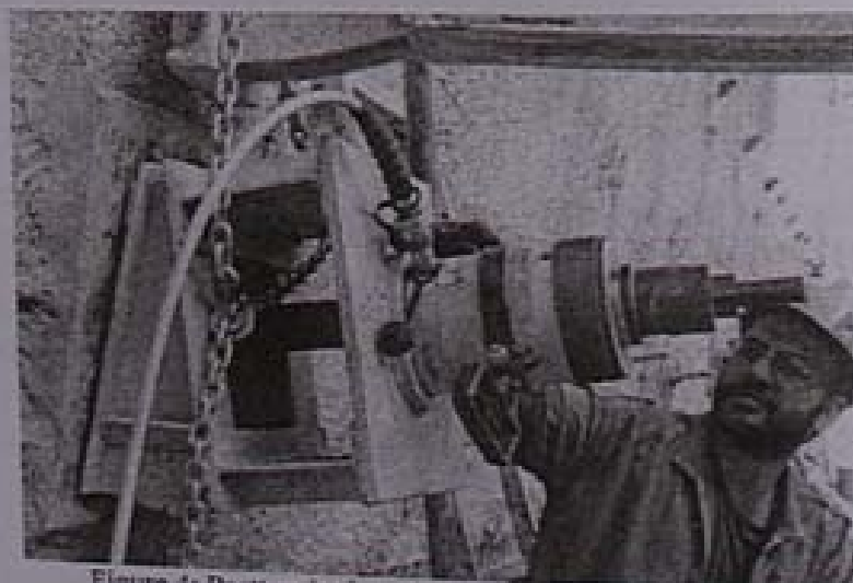
Figure 4: Posttensioning of anchors using hydraulic jack
